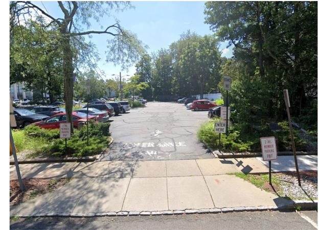
A section of pervious pavement can be installed in the parking lot to capture and infiltrate stormwater runoff from the parking lot. A preliminary soil assessment suggests that more soil testing would be required before determining the soil's suitability for green infrastructure.
