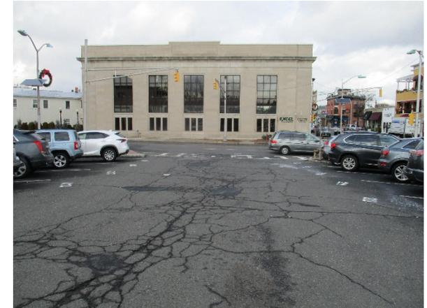
Downspout planter boxes can be installed at the station building to capture and store stormwater runoff from the roof. Additionally, lot #2 can be outfitted with pervious pavement to aid in the infiltration and capture of stormwater runoff. Tree filter boxes can be installed in the islands of lot #8 to capture runoff from the lot. A preliminary soil assessment suggests that more soil testing would be required before determining the soil's suitability for green infrastructure.
