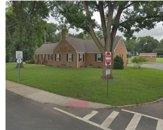
A rain garden can be installed along the building to capture stormwater runoff from the building's rooftop. Additionally pervious pavement can be installed in the parking lot to aid in stormwater capture and infiltration from the adjacent parking lot. A preliminary soil assessment suggests that more soil testing would be required before determining the soil's suitability for green infrastructure.
